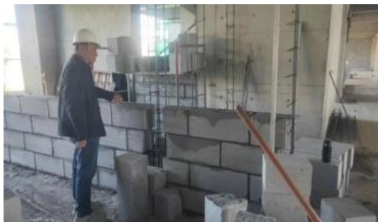
图8 砌筑施工监理验收
