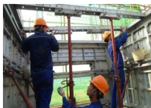
图9 楼面C槽、底龙骨安装
