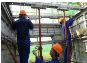
图9 楼面C槽、底龙骨安装
