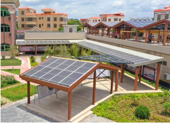
Figure 7 Overall construction effect of photovoltaic sun pavilions and rural housing facade improvement
