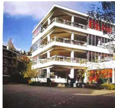
Figure 5 External view of Amsterdam Open Air School
