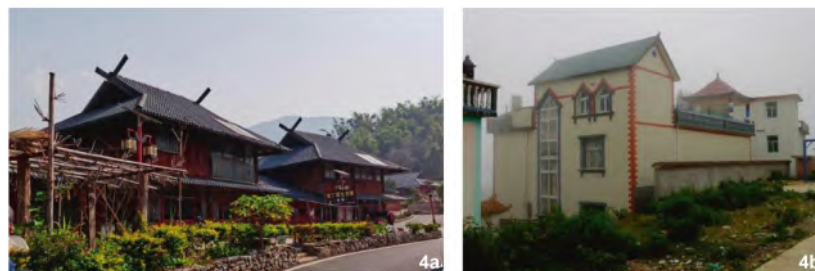
Figure 4 Two conditions of current new rural dwellings (4a: Well-constructed unified housing; 4b: Self-built housing that detracts from environmental character)
