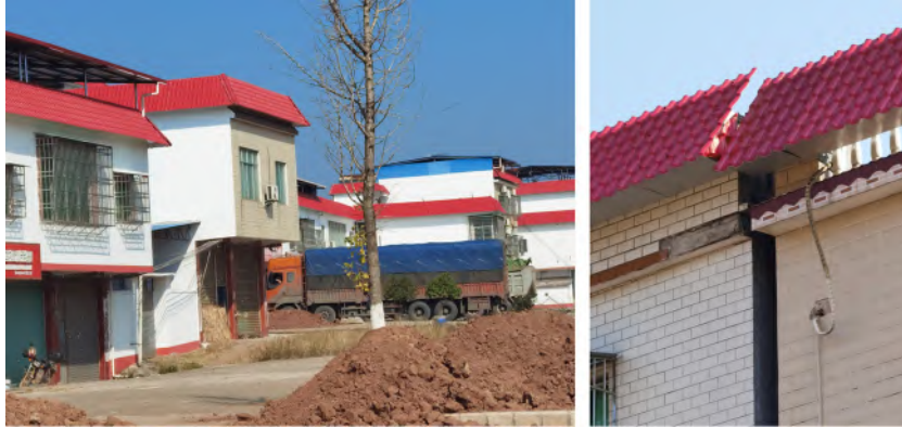
Figure 4 The lack of guidance in “flat-to-sloping” roof conversion practices does not yield satisfactory results in aesthetics and safety
