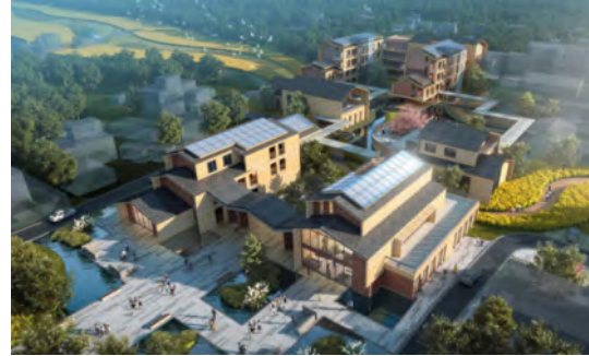
Figure 12 Photovoltaic building-integrated design of the Changshi Village Talent Station in Shaoguan City
