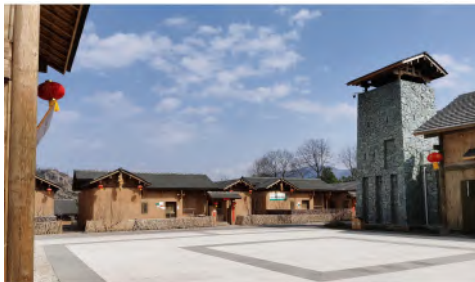
Figure 8 Interior view of Point No. 2 in Sanhe New Village, Zhaojue County, Sichuan
