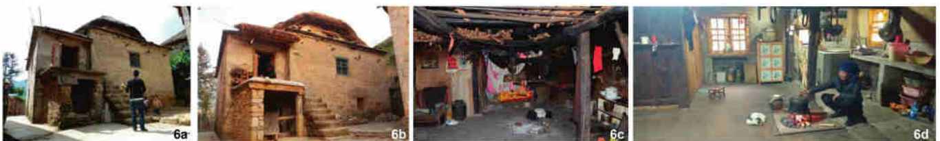
Figure 6 Conservation and restoration of Hani mushroom houses in Azheke Village, Yuanyang
