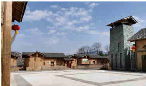
Figure 8 Interior view of Point No. 2 in Sanhe New Village, Zhaojue County, Sichuan
