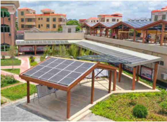
Figure 7 Overall construction effect of photovoltaic sun pavilions and rural housing facade improvement
