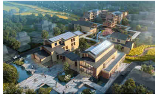
Figure 12 Photovoltaic building-integrated design of the Changshi Village Talent Station in Shaoguan City
