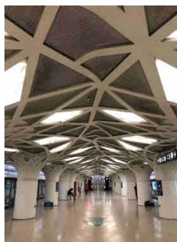
Figure 9 Lighting facilities at Forest Park subway station
