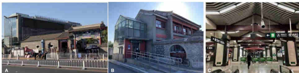
Figure 7 A, B, and C: Entrance/Exit and interior space design of Nanluoguxiang Subway Station
