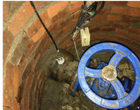
Fig.6 Place sensors downhole
