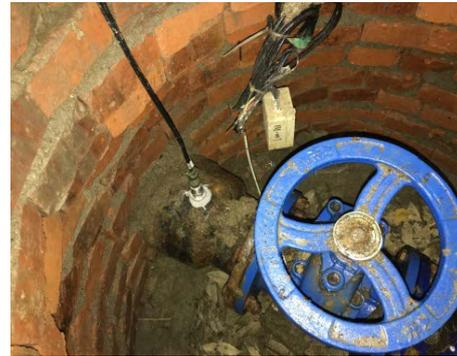
Fig.6 Place sensors downhole
